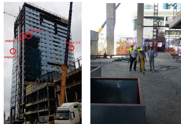
Figure 18 Reflective marks at the 15th floor During monitoring work
