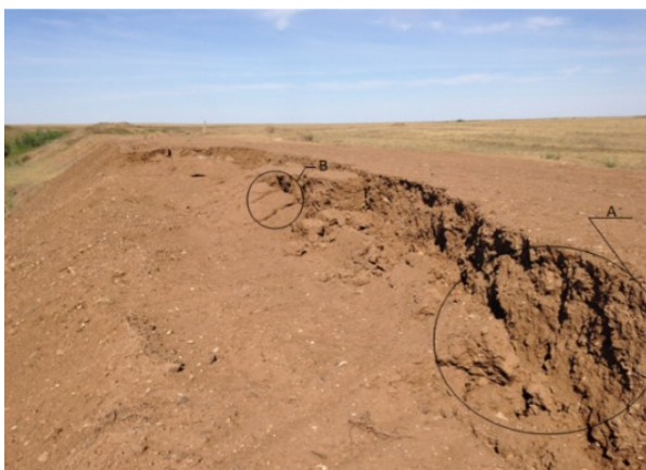
Figure 9 Land sliding of the dam investigation
