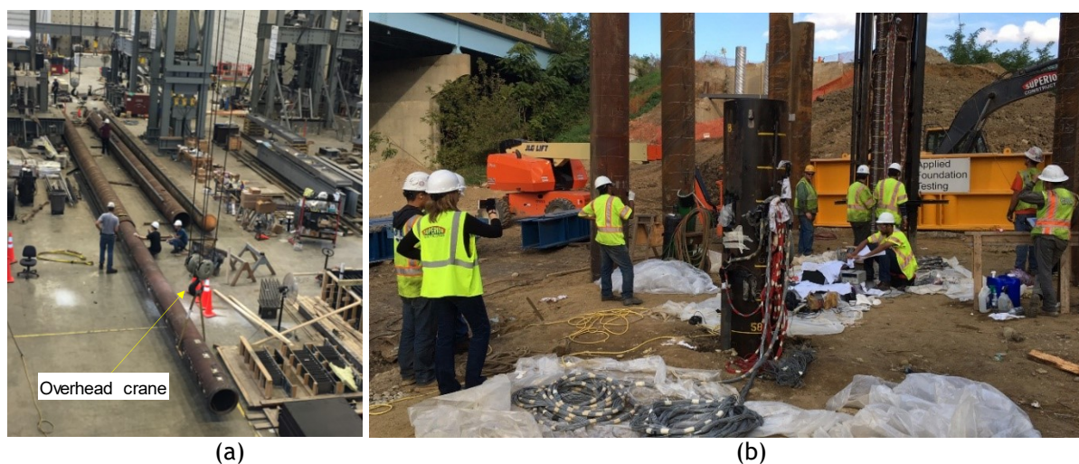
Figure 9. Static and dynamic load tests on large-diameter open-ended pipe pile: (a) assembly of the double-wall system; (b) on-site operations at the end of pile installation;
