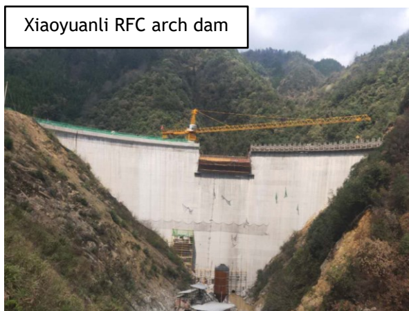
Figure 2. Some examples of RFC arch dams during construction
