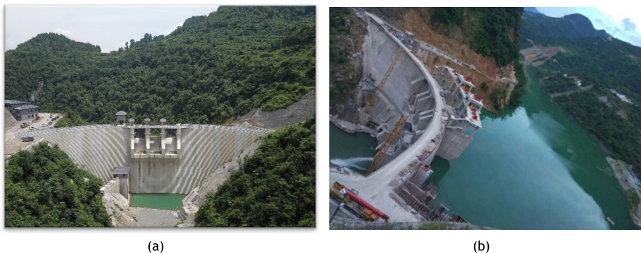
Figure 1. Notable examples of completed RFC arch dams; (a) Lyutang RFC arch dam in Guizhou Province; (b) Baijia RFC double curvature arch dam in Shaanxi Province
